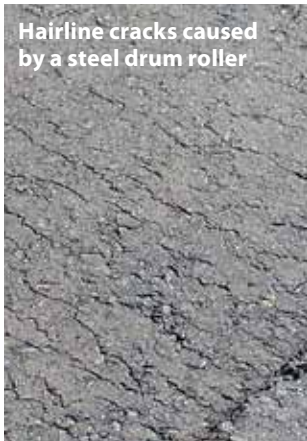
Fig 4. Remove hairline cracks from HMA pavement
