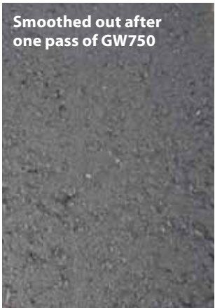
Fig 4. Remove hairline cracks from HMA pavement
